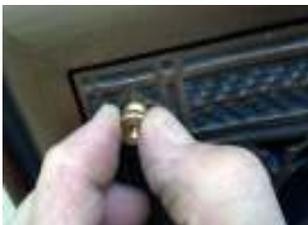
**FINALLY:** If installed in the winter months use the **Plug Plate** to block cold air from entering the foundation. If installed in any other season install the **Fiberglass Screen Plate** for ventilation purposes. In either case, complete the installation by re-placing the **Foundation Vent** Up-Right according to the sticker, and secure by snugging up the four **Knurled Knobs**.
