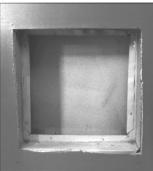
Clean dust from plenum or duct with a damp rag and some house cleaner like 409.
