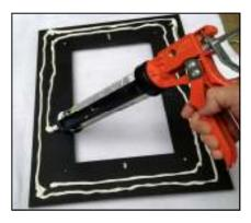
THIRD VERY IMPORTANT: apply clear Adhesive Caulk (not included) to the back of the Base-Frame. The Adhesive Caulk will provide a water seal to prevent rain water from getting into your foundation plus will help secure the Base-Frame to the Foundation for years to come. Apply two thick continuous (1/4" to 3/8") beads all the way around the back of the Base-Frame about 1/2" and 1"from the outside. Adhesive Caulk ( without silicone) is available at any Hardware store or Home Depot or Lowes
