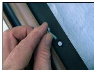
**Step 2:** Insert the 3/4" Stainless Steel Bolts into the two countersunk holes in the front of the Base-Frame. Then insert and tighten the two Continuation Nuts to the Bolts protruding through the back of the Base-Frame, tighten until snug.
